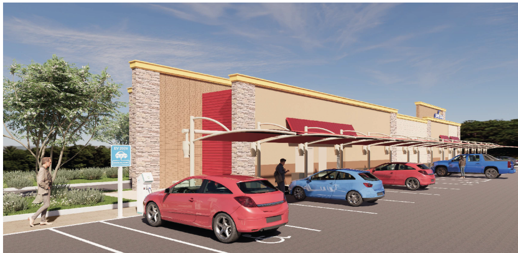
View 3: Inside the Project Site, near the eastern border, looking southwest at the northern aisle of vacuum stations.
